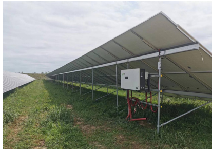
Slovenia | 6MW Ground PV EPC Project
