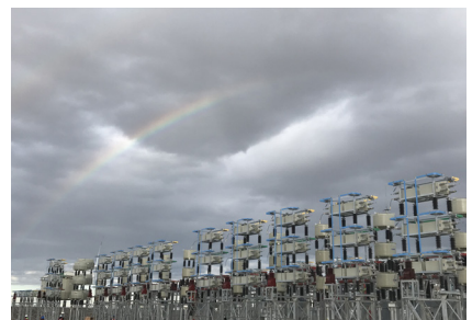
Mexico | Amistad I-IV Station, Magdalena Station and Dolores Station Power Quality Project
